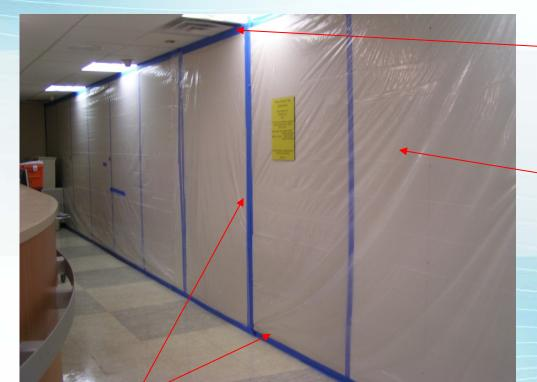
Sealed with cloth tape (on all edges of hoarding) – ensure air tightness NUH \*subject to above ceiling site work/constraint Noncombustible hoarding up to false ceiling
